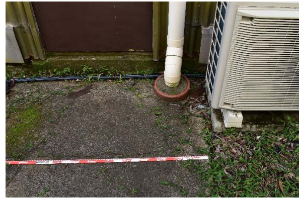
Figure 23: Evidence of sub-surface disturbance due to service installation
