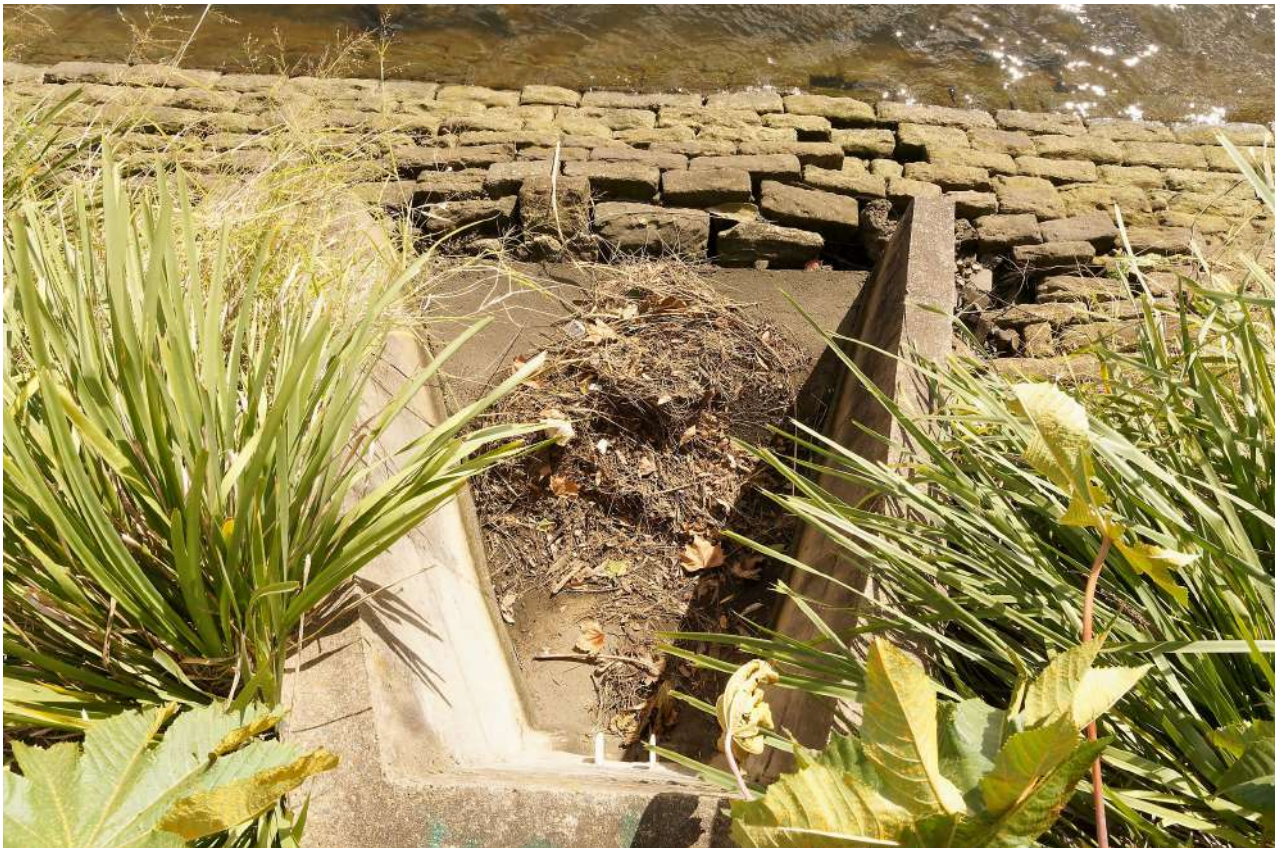
Large concrete outlet in eastern sandstone wall.
