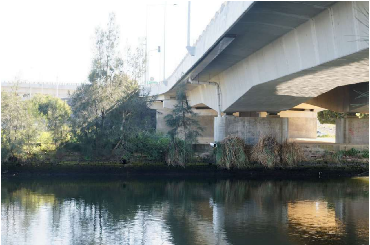
OP1 – 10 m south west of bridge (WestConnex ramps)
