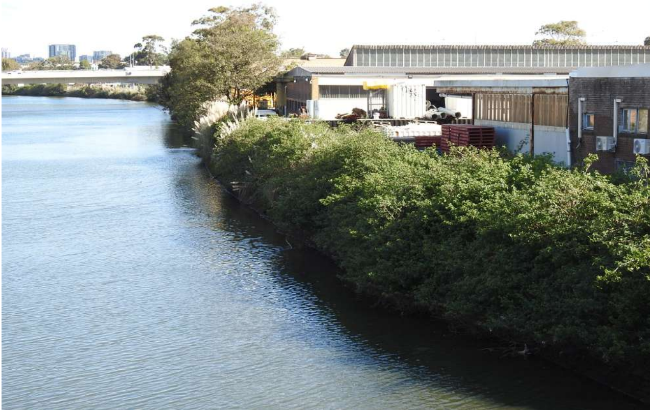
OP23 – taken from Campbell Road Bridge looking west
