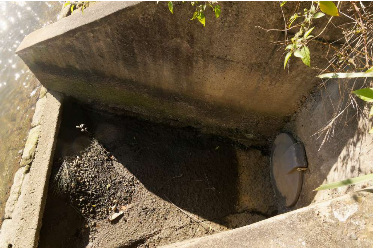
Large concrete drain
