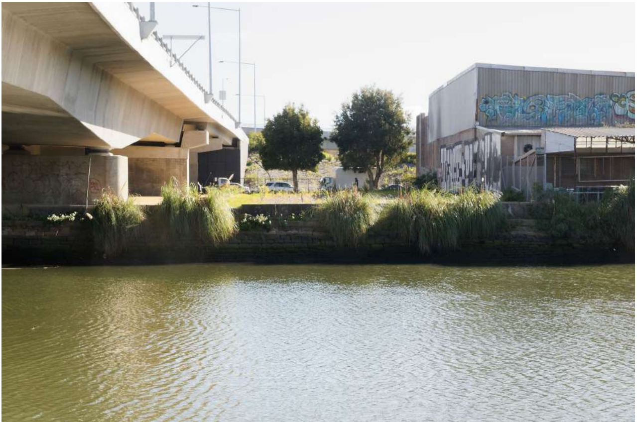
OP2 – 5 m north east of bridge
