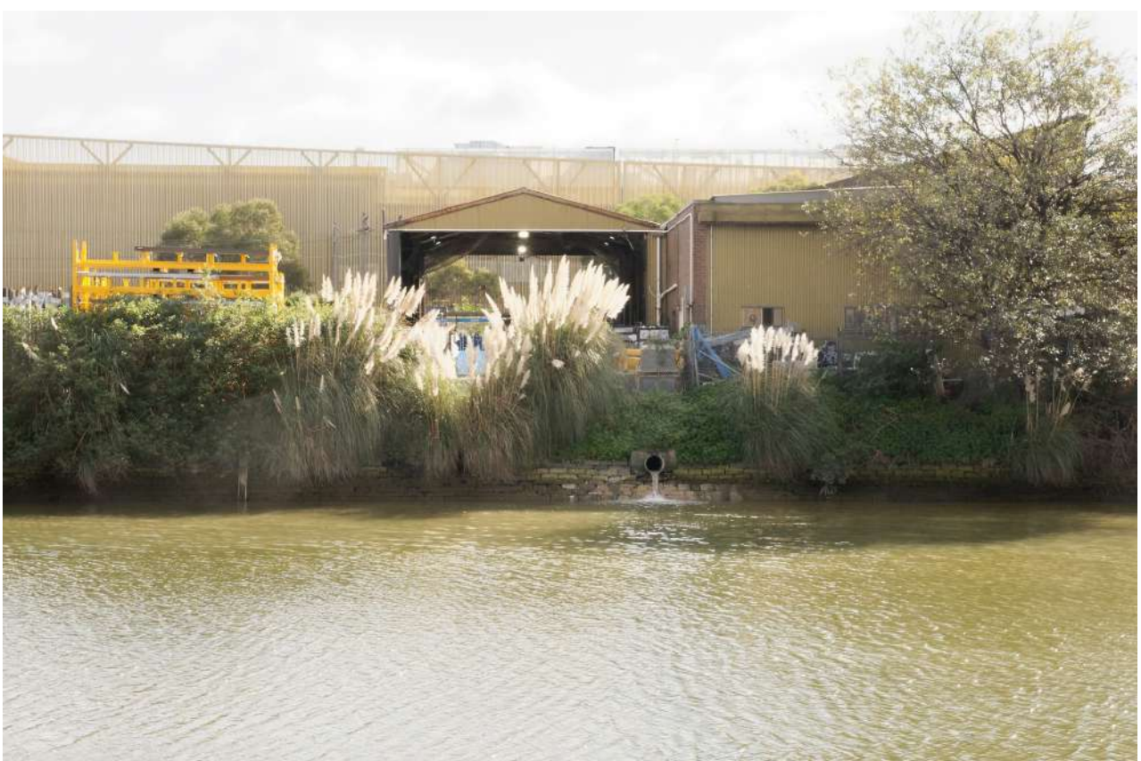
OP15 – 260 m north east of bridge: looking to 32 Burrows Road
