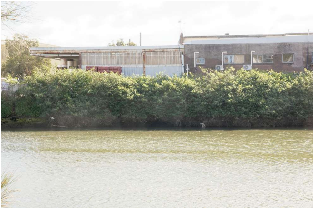
OP21 – 380 m north east of bridge; looking to 32 Burrows Road
