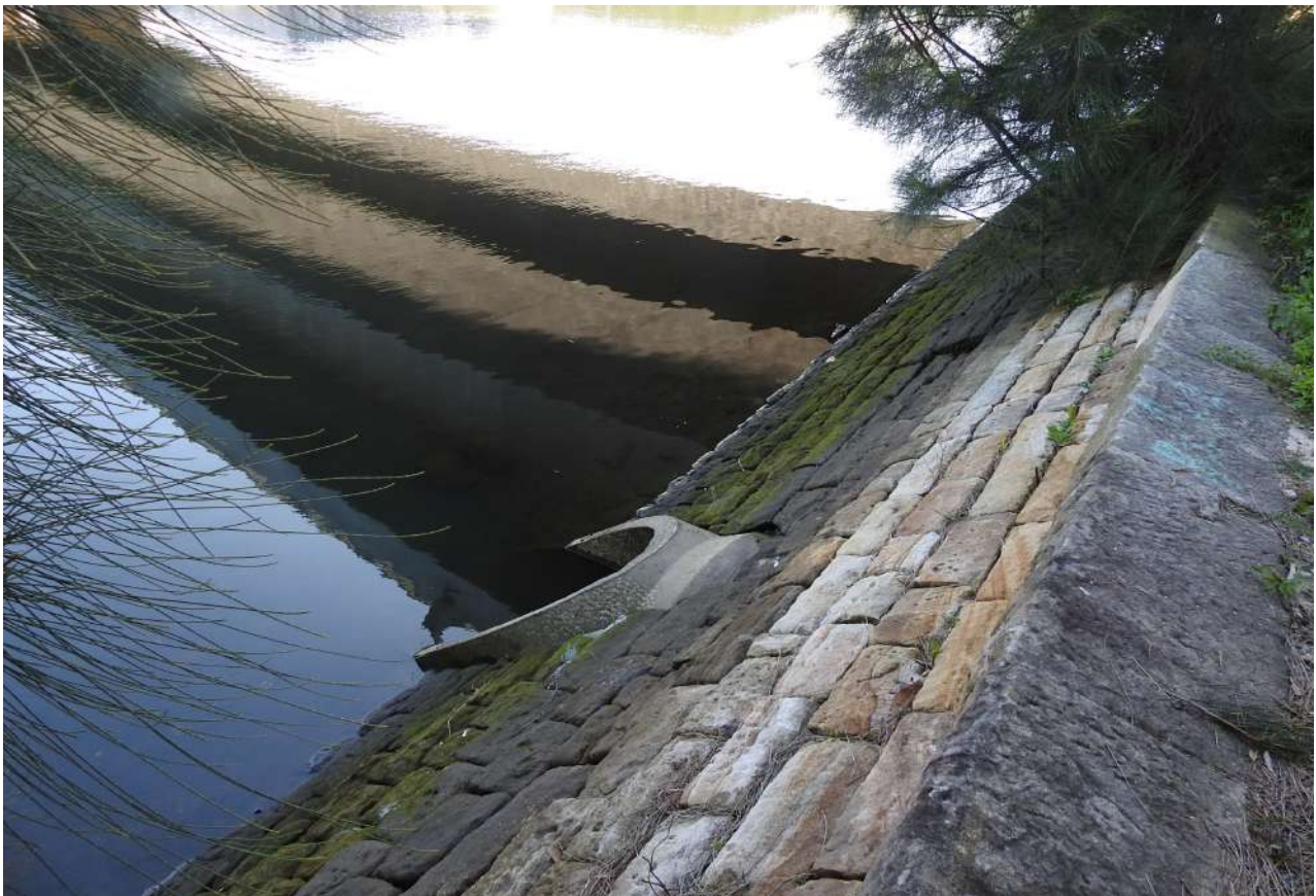
Drain in sandstone wall
