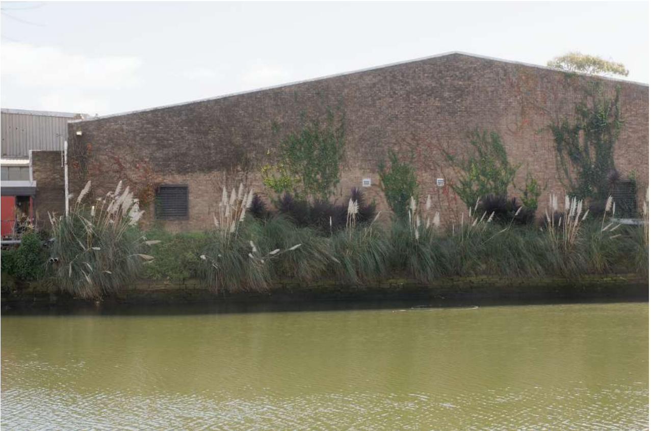
OP4 – 40 m north east of bridge
