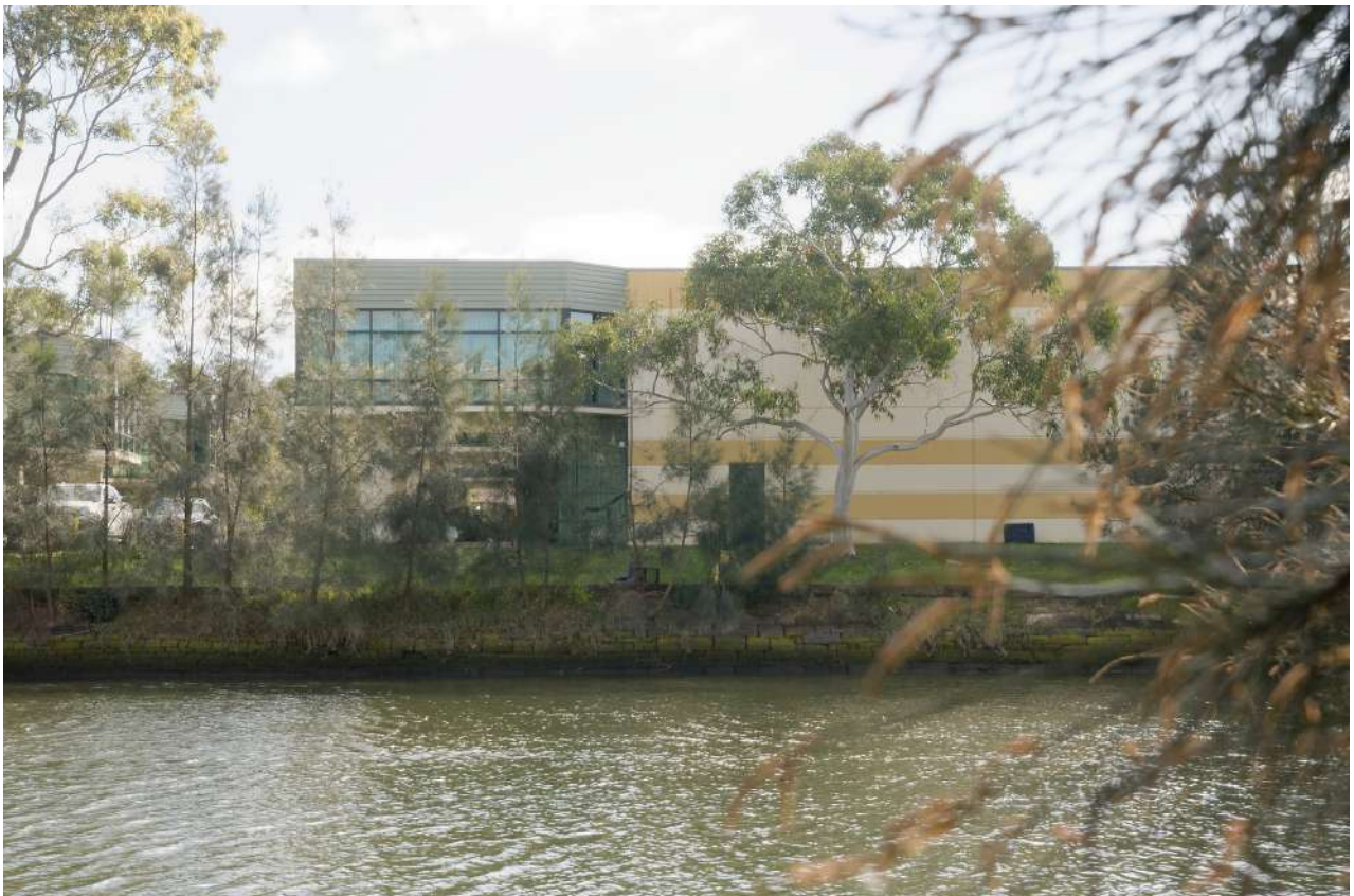
OP8 – 120 m north east of bridge: looking to central part of 24-26 Burrows Road
