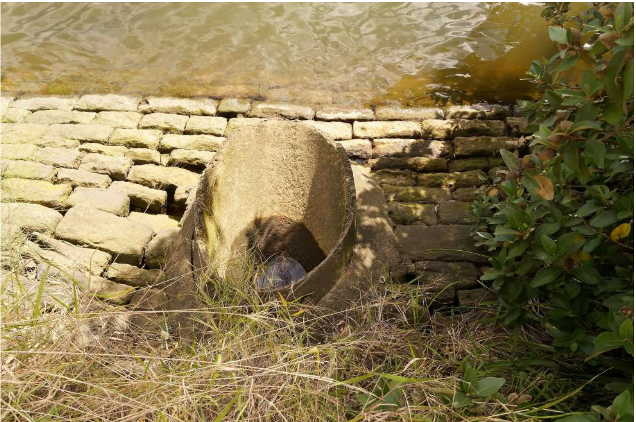
Small concrete pipe in eastern sandstone wall
