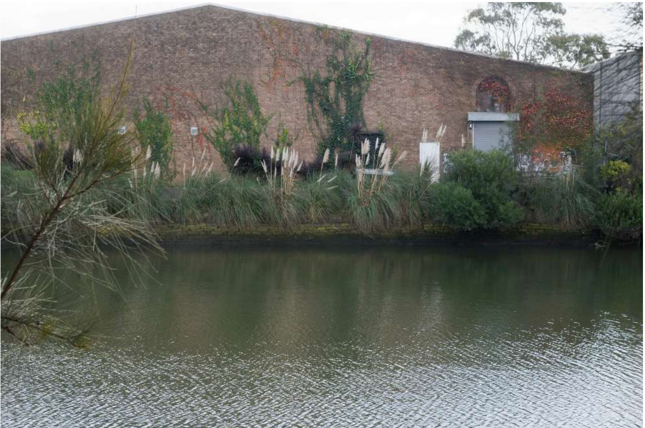
OP5 – 60 m north east of bridge: looking to 22 Burrows Road
