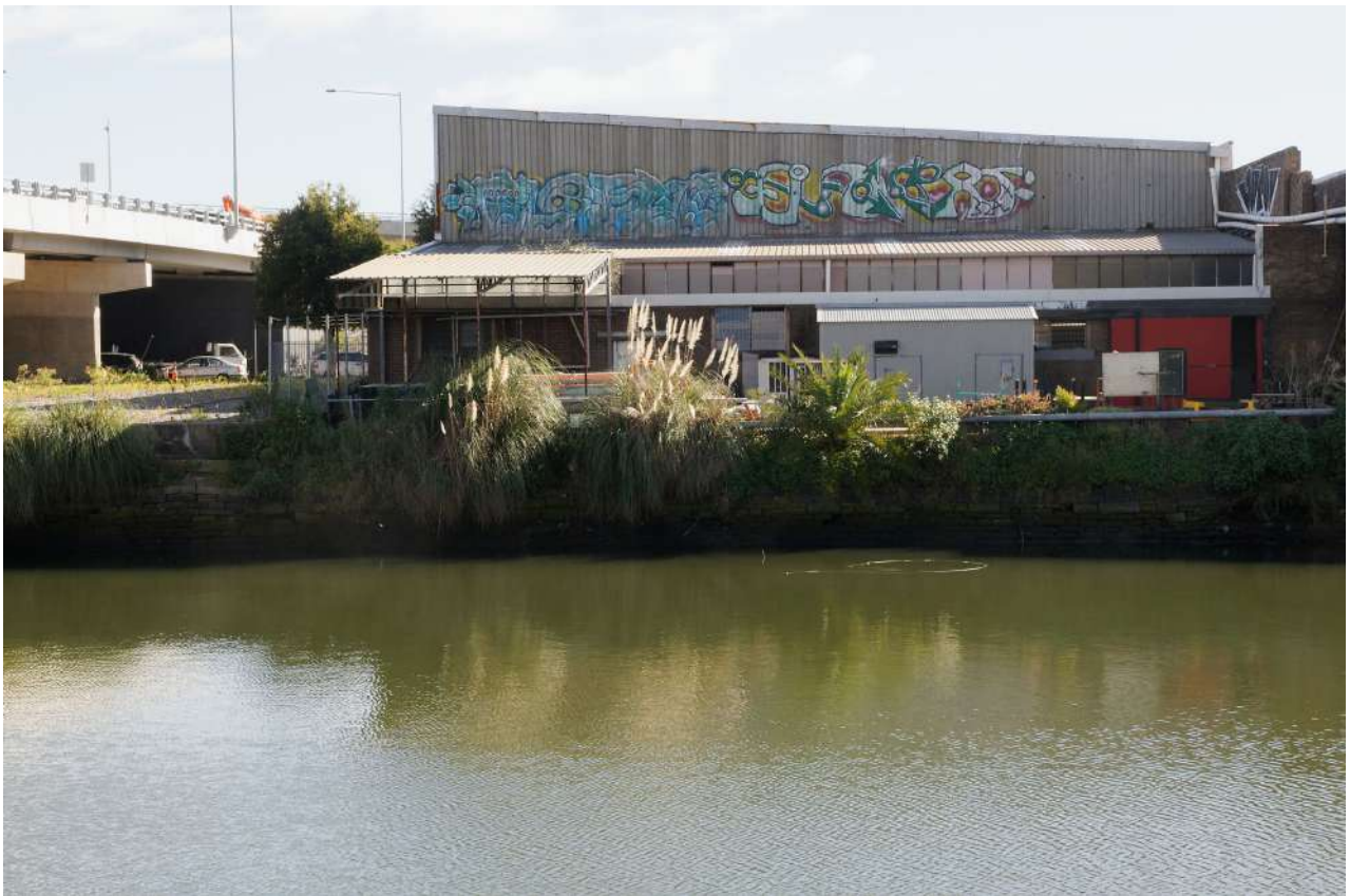
OP3 – 20 m north east of bridge
