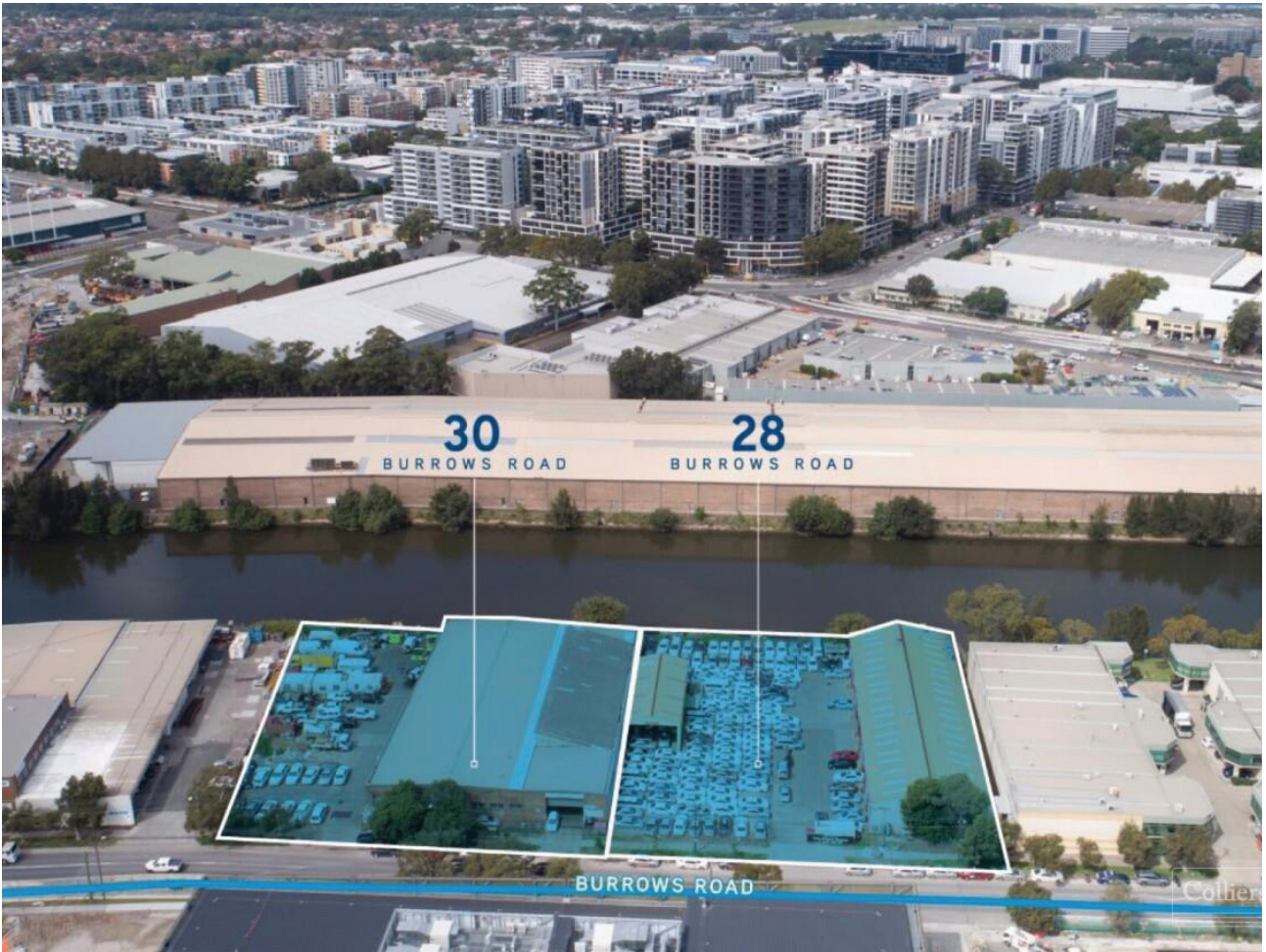
EXISTING BUILDINGS AERIAL VIEW FROM BURROWS ROAD
