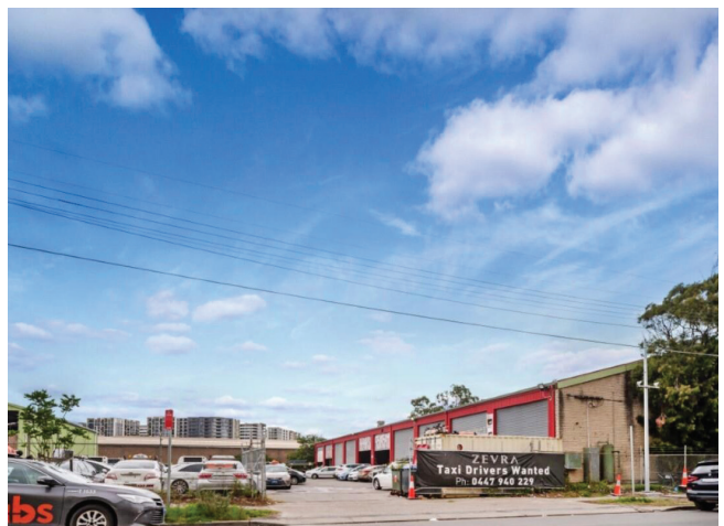
EXISTING NORTHERN WAREHOUSE FACADE VIEW FROM BURROWS ROAD
