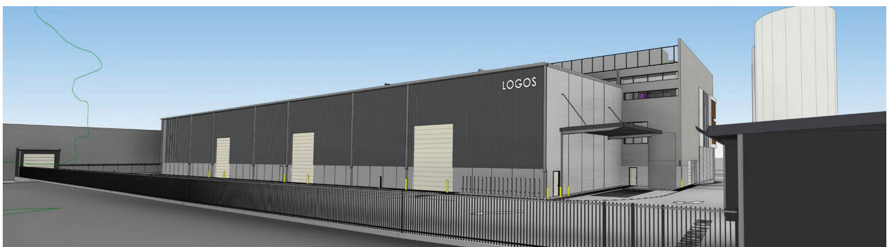
SOUTH EASTERN CORNER FRONTING ALEXANDRA CANAL
