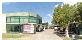
(3) Industrial Strata Units
