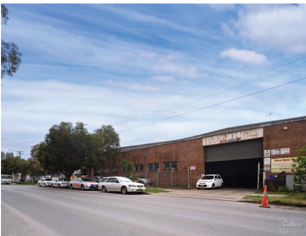
EXISTING NORTHERN FACADE - VIEW FROM BURROWS ROAD
